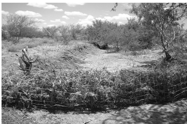
Fig. 2. Wire and Branch Dam
