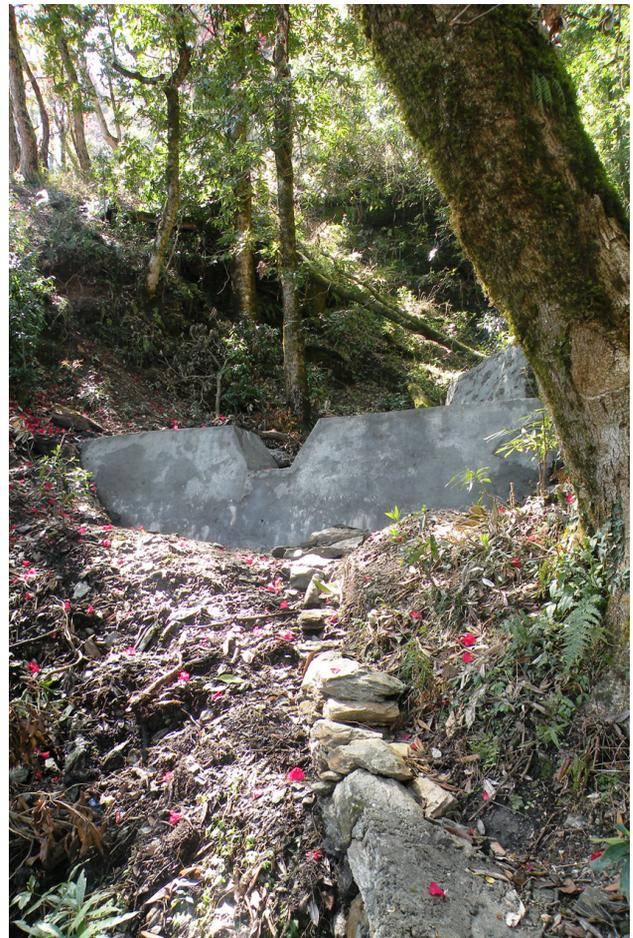
Fig. 8. Debris dam to check gully erosion in forest land
