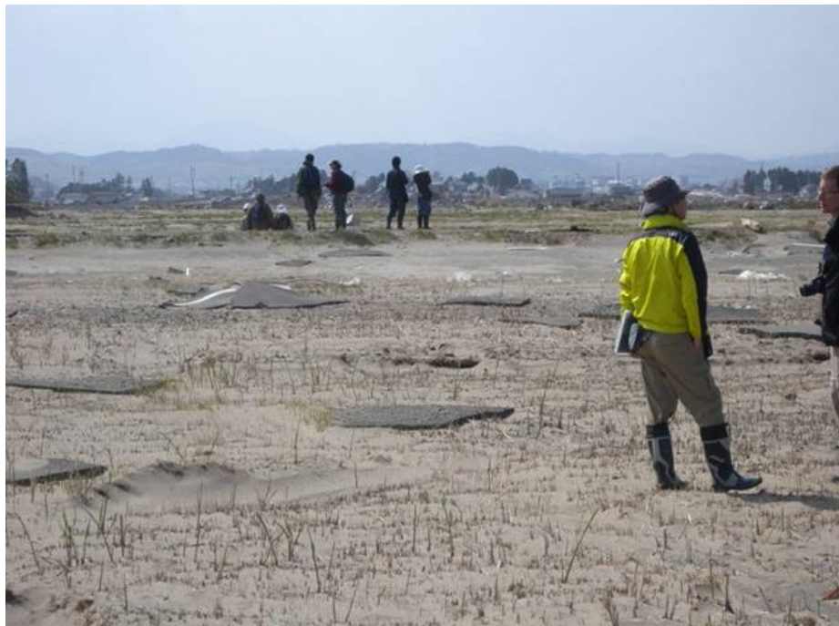
Figure 11. Asphalt from the road in tsunami deposit.
