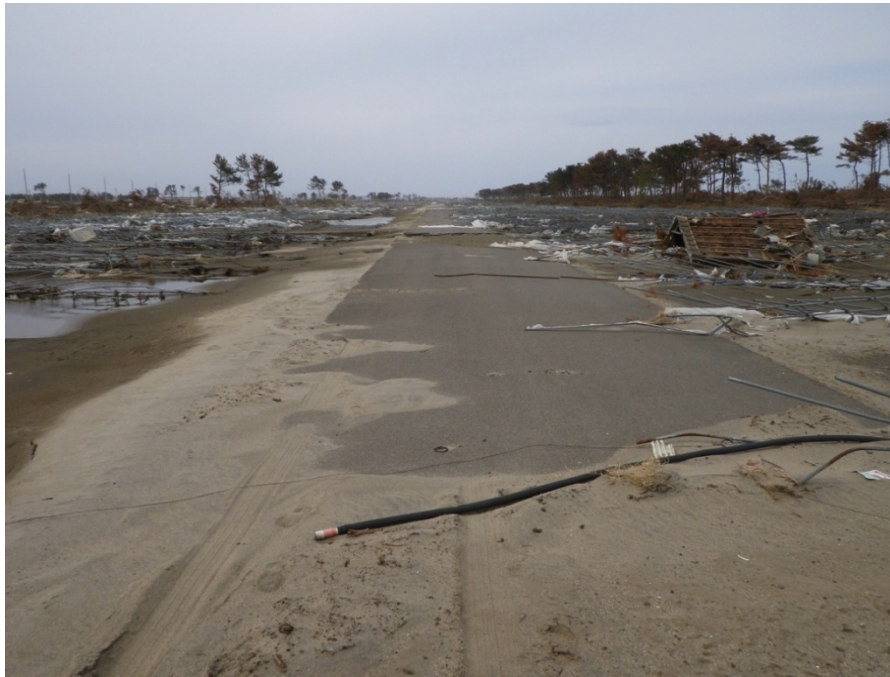
Figure 9. Remains of greenhouses north of site 3-10 (450 m from shore, Natori City). According to interviews, the surface of the farmland was at about the same level as the road prior to the tsunami, but erosion during the tsunami removed sediment from the farmland resulting in the elevation difference apparent in the photograph.
