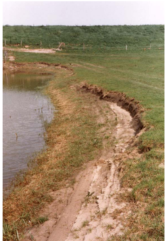
Fig. 10. “Cliff” in the wall of the “canal” formed due to erosion by an “upstream” current from left (=west) to right (=east).
